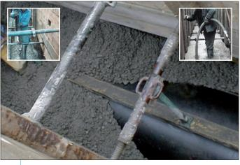
*Installation of the buoyancy control* and the front formwork, application of the release agent
