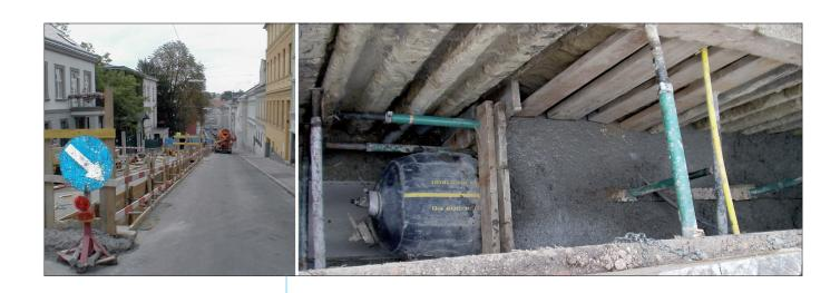
The **advantages of the egg-profile** in sewage technology are generally known. Sewer structures in cast-in-place concrete are highly valued because of their outstanding quality, tightness and durability.
