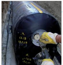
${\it Installation of the pneum form:}$ inflating by means of construction compressor
