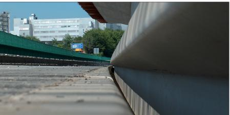
**Polymer concrete** is a perfect material for civil engineering purposes: Its high strengths enable the construction of very slim components; its **chemical stability** makes it resistant to aggressive media. The non-porous and hydraulically smooth surface ensures that it is 100% corrosion-free. Constructions made of polymer concrete are characterised by longevity and ensure an investment's sustainability.
